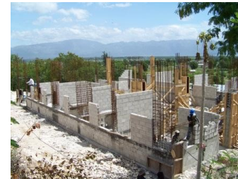
Back of the Health Center looking northwest
