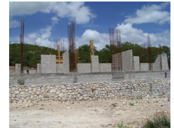
West side of the building looking east
